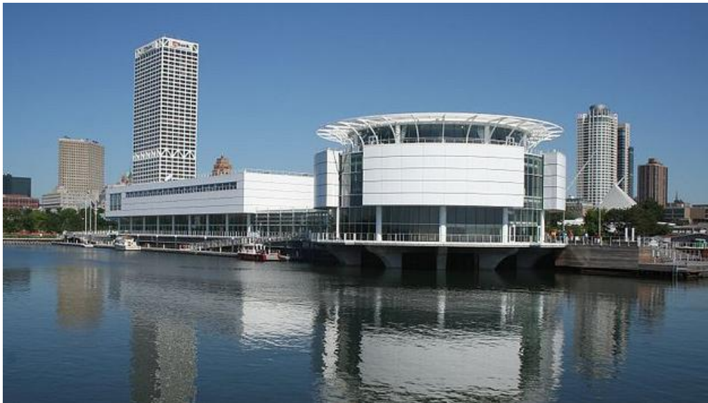
Figure 33 – Pier Wisconsin, Photo consent of Robert Powers
